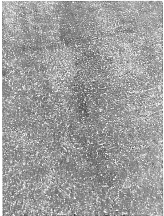
Photo 25: Typical Jet Seal on Apron I
