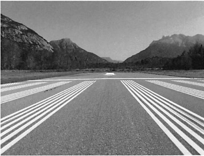
Photo 14: Displaced Threshold for Runway 23
