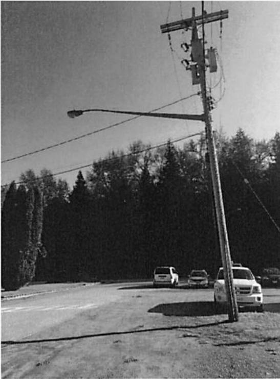
Photo 39: Terminal Exit Road and Parking
