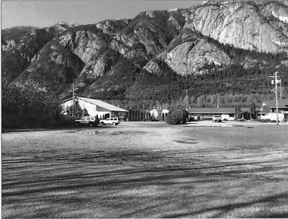
Photo 45: Settlement and Ponding in Gravel Parking Area
