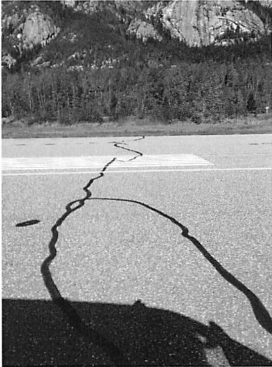
Photo 11: Sealed Transverse Crack
