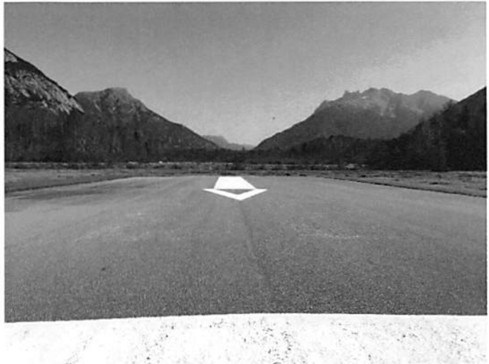
Photo 15: Displaced Threshold for Runway 23
