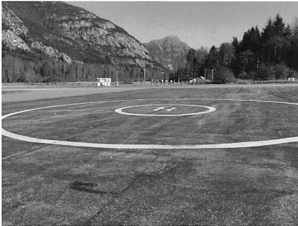
Photo 23: Apron Helicopter Touchdown Pad on Apron I
