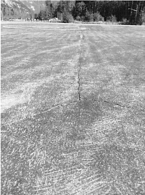
Photo 26: Typical Jet Seal on Apron I
