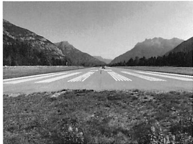
View to East
